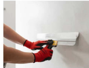
Internal Finish: Putty finish over plaster on the walls and ceiling
